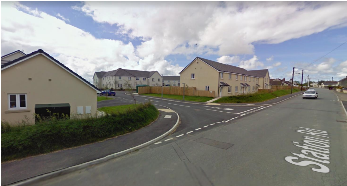
View of 23 Station Road facing South West into Phase 1
