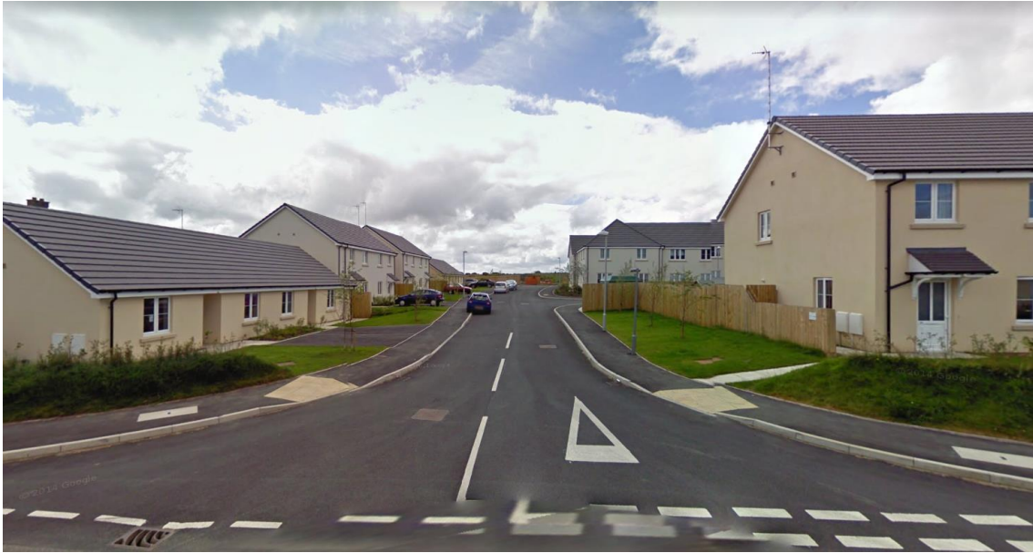
View of access road looking South East, existing Phase 1 development
