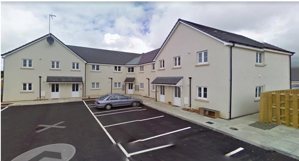
View looking North to adjacent phase 1 from Site
