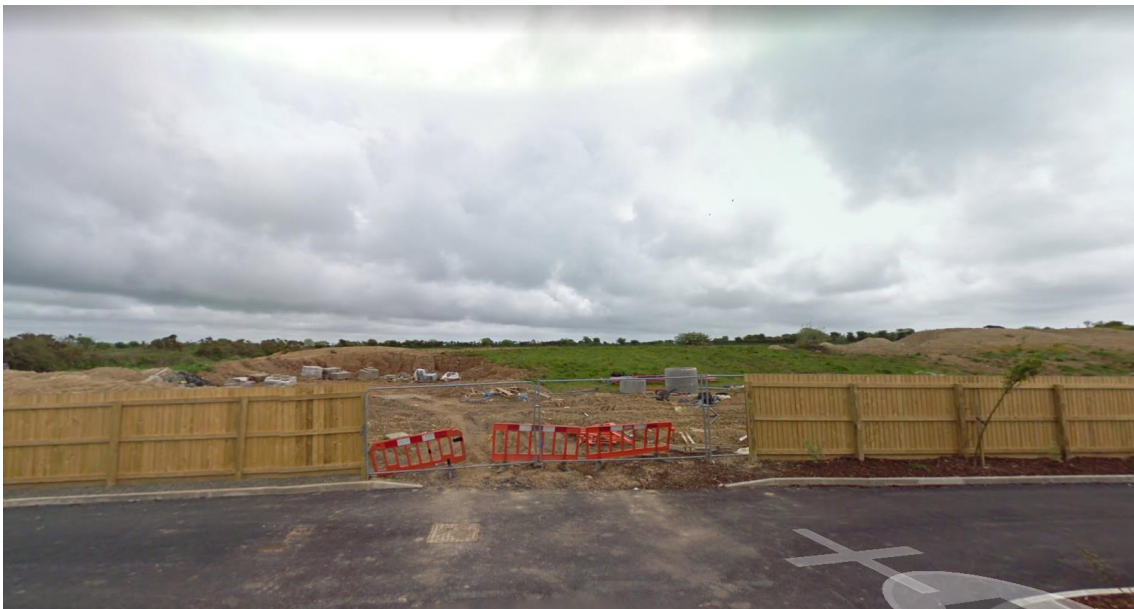
View looking onto site, evidence of previous drainage components from Phase 1
