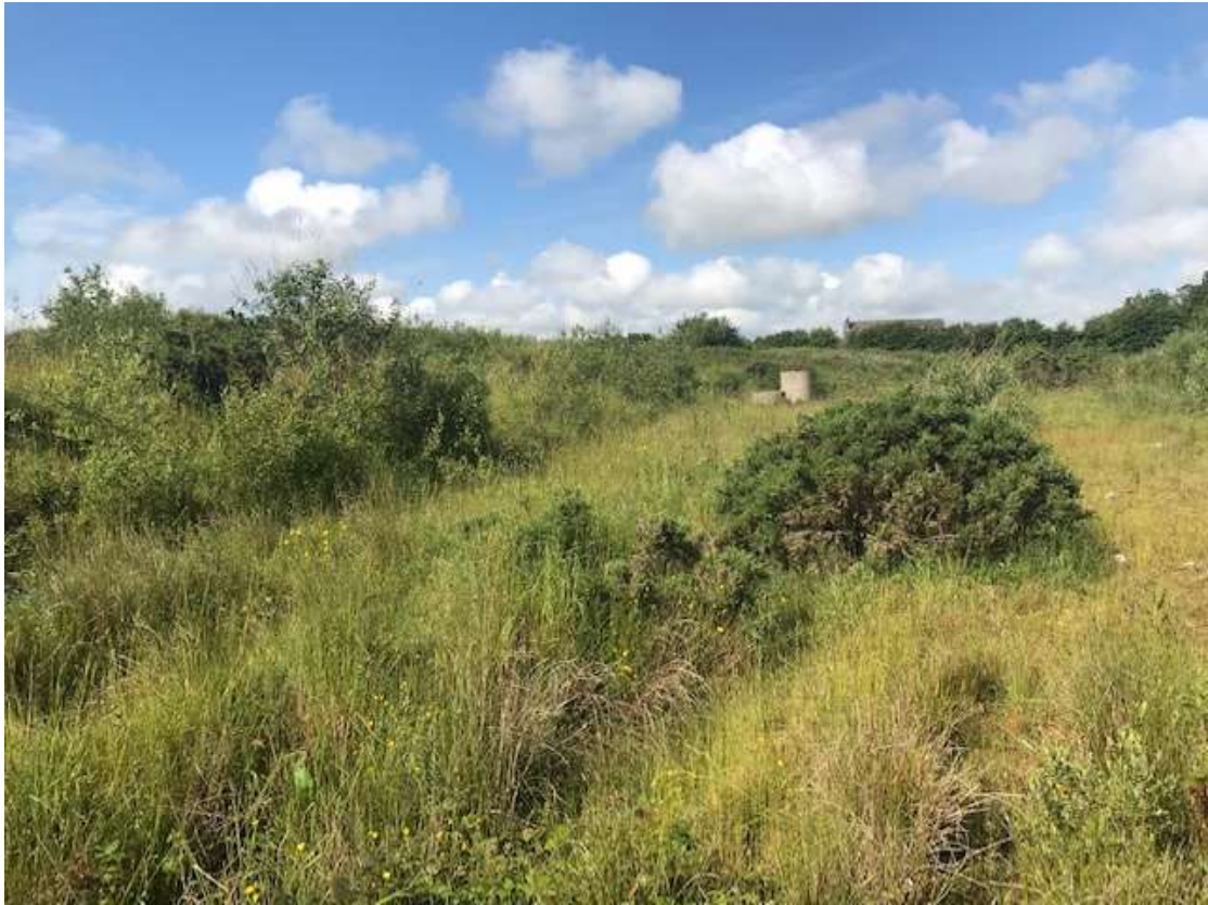
Photo 3: View west along the base of a spoil heap where a deeper channel was still visible containing concrete inspection chamber pieces
