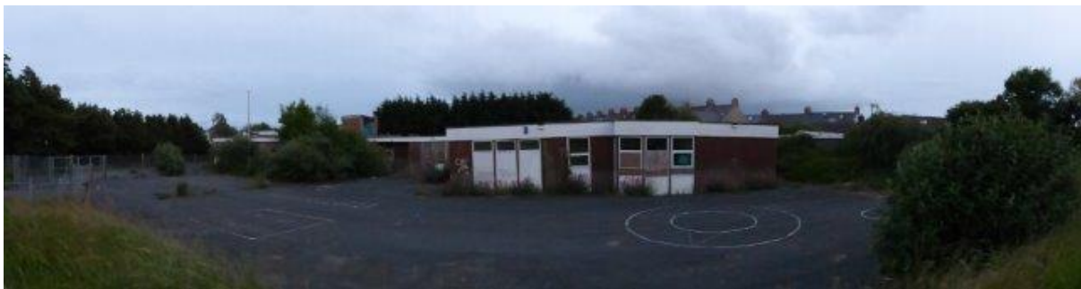
Figure 4 - Building North side
