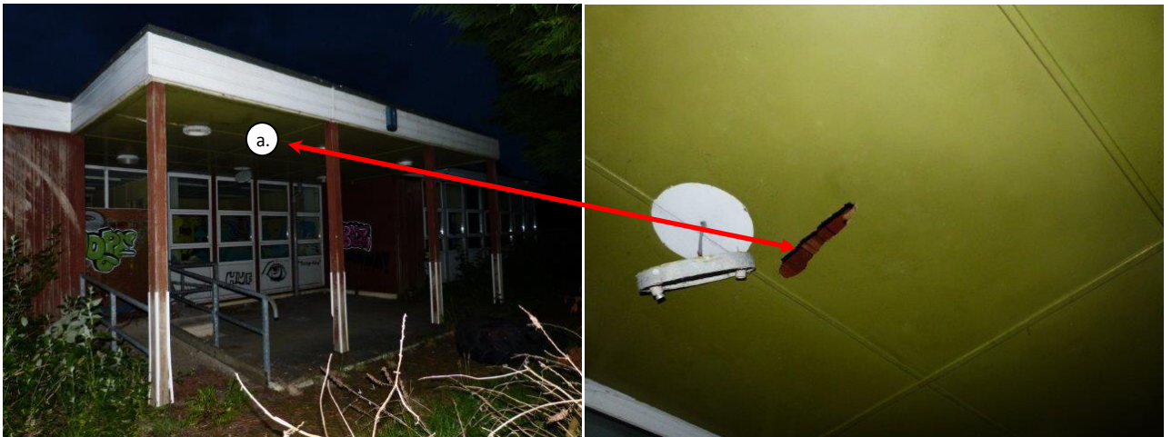
Figure 4 - South West – southern entrance porch
