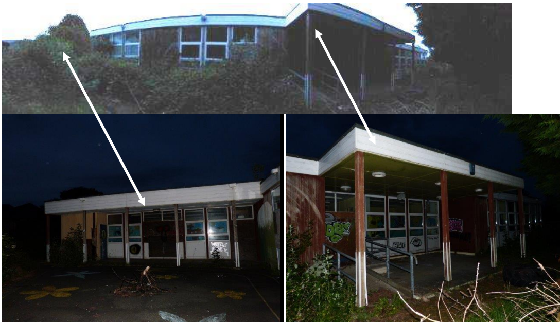
Figure 3 - Building West side
