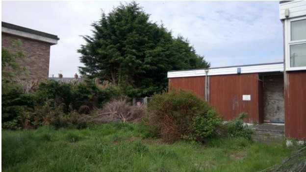
Figure 1 - Building south east corner looking south
