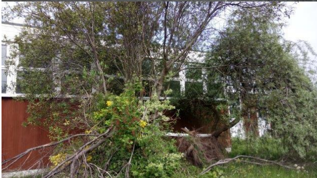
Figure 2 - Building South side
