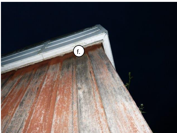
Figure 8 - South side on corner near entrance – not a PAP but tight fascias
