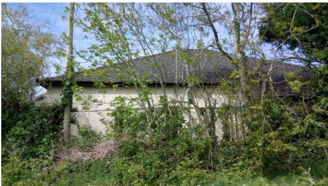
i. North west corner of the site
