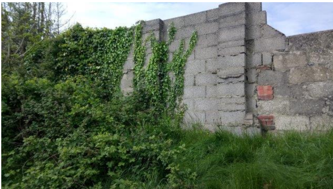
h. Area of wall on the west boundary with ivy
