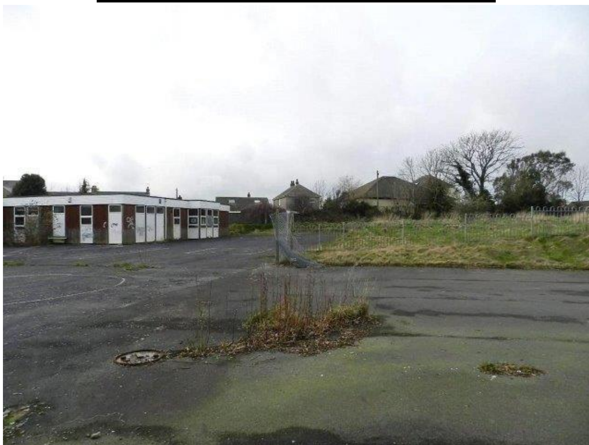
Overgrown playground area and old school buildings with tarmac car park area
