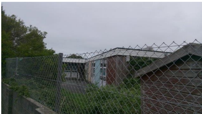
West side of school looking north
