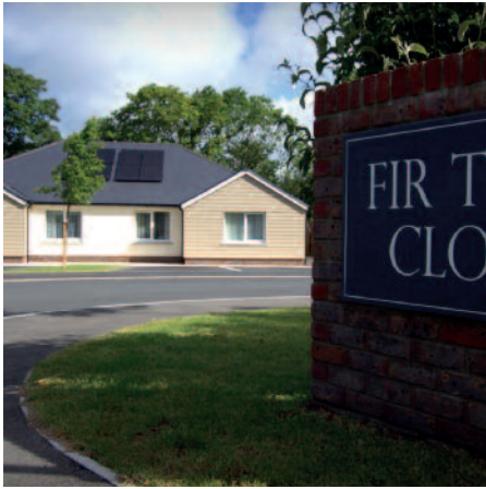
Fir Tree Close, Merlins Bridge.
