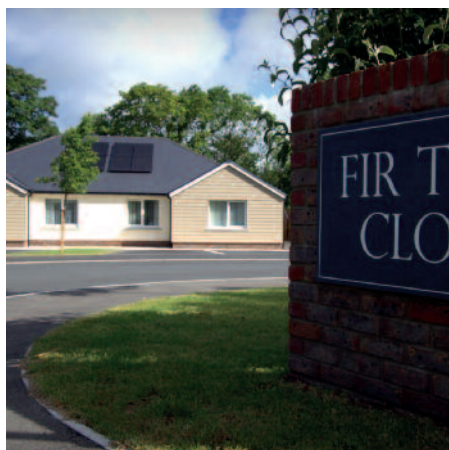
Fir Tree Close, Merlins Bridge.
